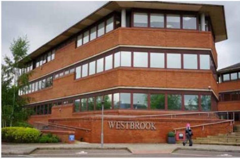
2. Existing ramp access and signage
