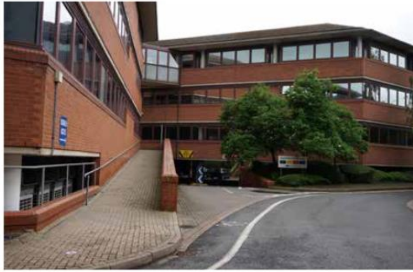
3. View into the undercroft parking and adjacent ramp access to ground floor
